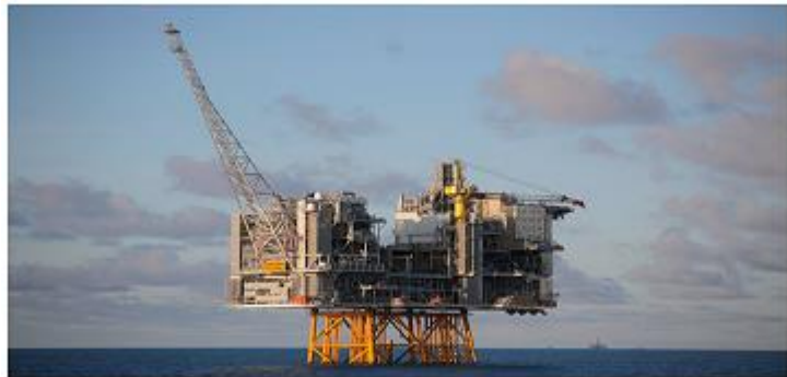
The Edvard Grieg platform has been successfully installed and commissioning is ongoing.
